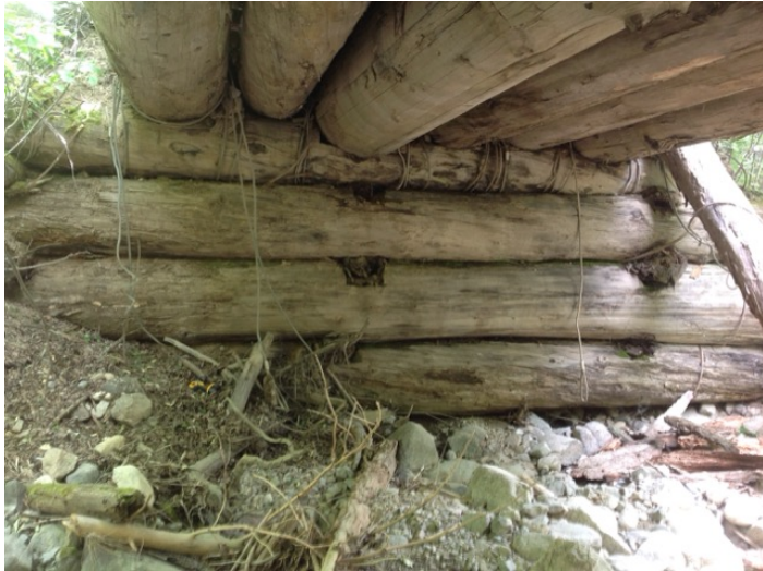
Left Bank Abutment when facing downstream
