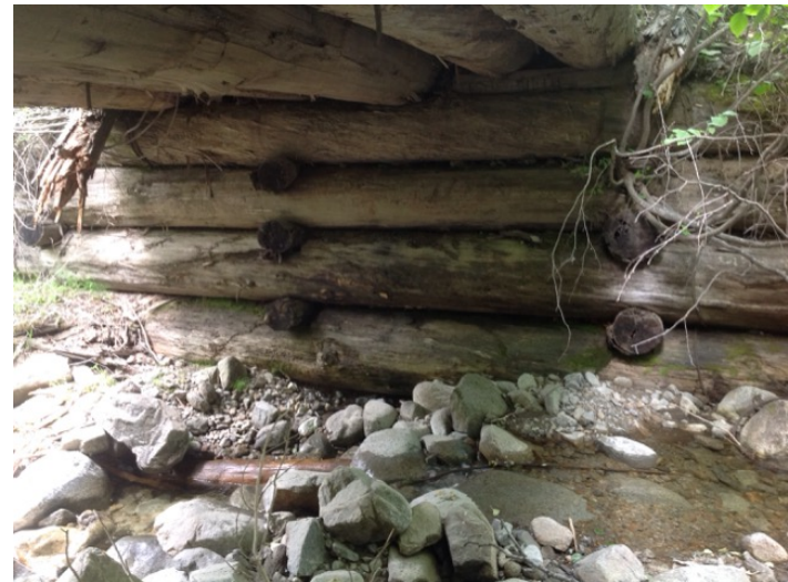
Right Bank Abutment when facing downstream
