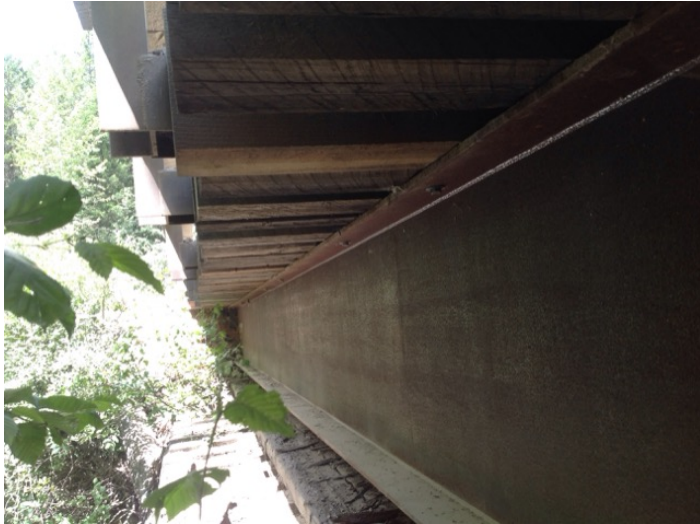
deck to girders bolts
